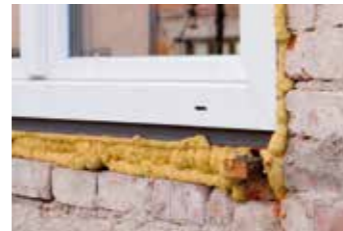
Examples of traditional sealing methods
